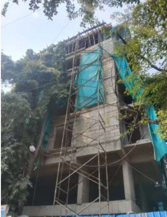
Terrace slab RCC work in progress.
