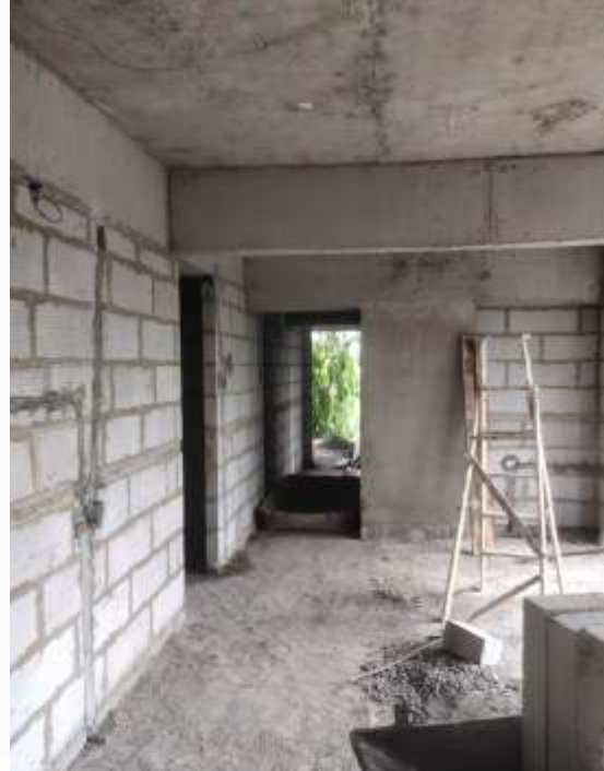
4 th floor blockwork in progress.
