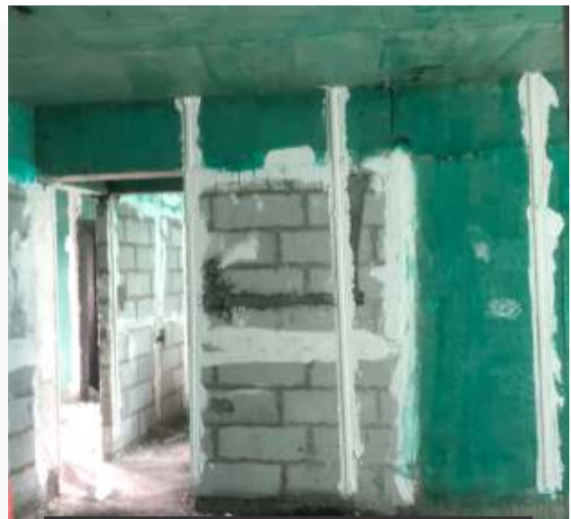
3 rd floor gypsum work in progress.
