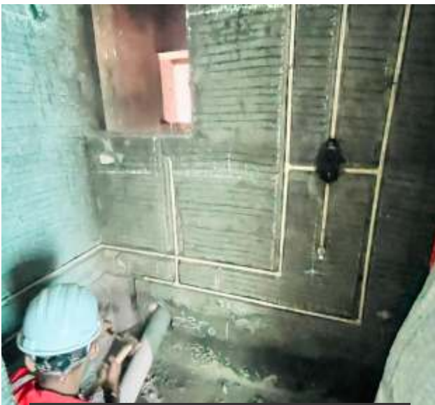
1 st floor concealed plumbing work in progress.
